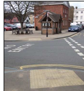
Dropped kerbs and tactile paving in Potton town centre
